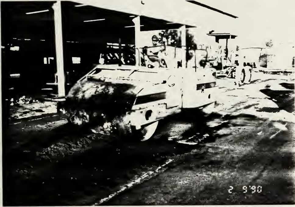
Figure 2.23 Vibratory Roller and Partial Slab View
